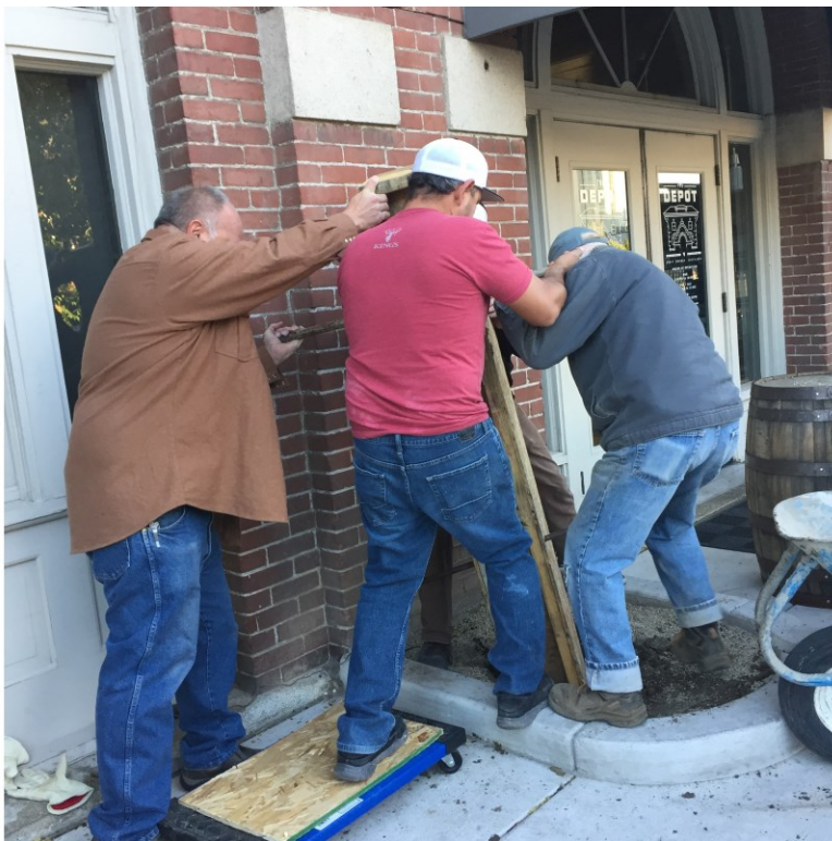
Gravel added to the bottom of the hole to provide moisture drainage. Scott, Jose, Michael Lopez of The Depot and Tom muscle up the very heavy marker in its cradle for insertion into the ground.
