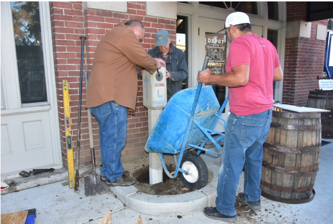
Adjusting the orientation of the marker and checking the plumb. Additional gravel is poured into the hole for drainage and to assist future marker removal if required.
