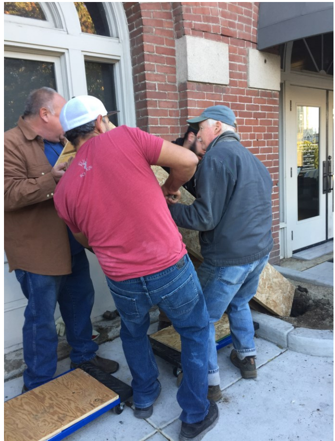
Gravel added to the bottom of the hole to provide moisture drainage. Scott, Jose, Michael Lopez of The Depot and Tom muscle up the very heavy marker in its cradle for insertion into the ground.
