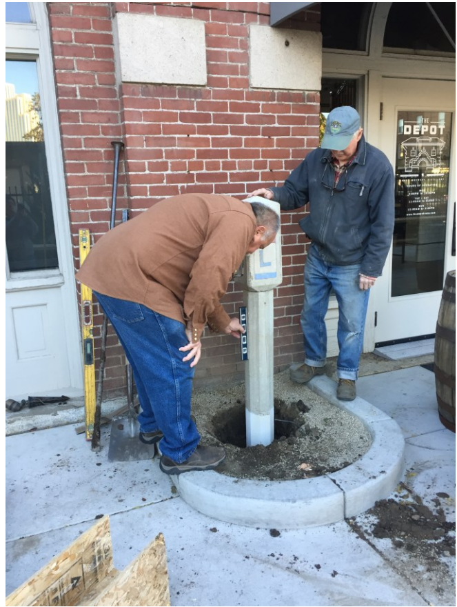
Adjusting the orientation of the marker and checking the plumb. Additional gravel is poured into the hole for drainage and to assist future marker removal if required.
