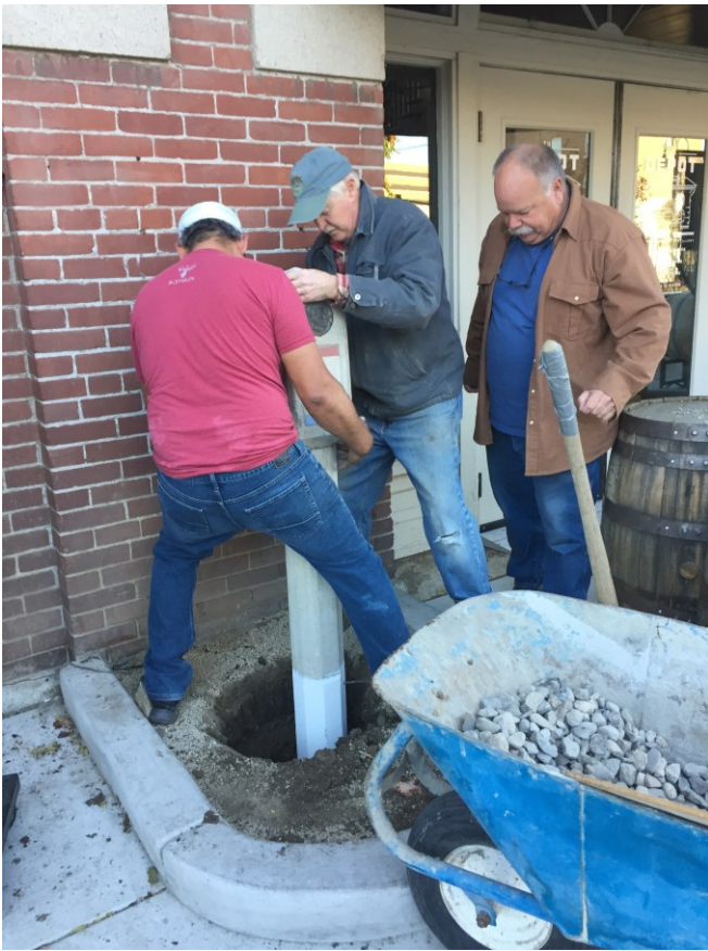
Adjusting the orientation of the marker and checking the plumb. Additional gravel is poured into the hole for drainage and to assist future marker removal if required.
