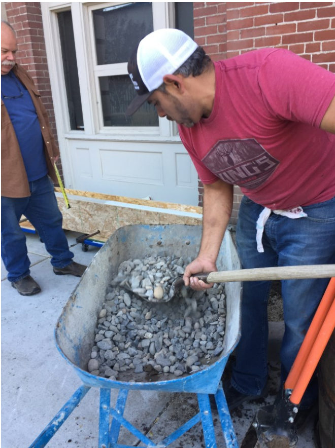
Gravel added to the bottom of the hole to provide moisture drainage. Scott, Jose, Michael Lopez of The Depot and Tom muscle up the very heavy marker in its cradle for insertion into the ground.
