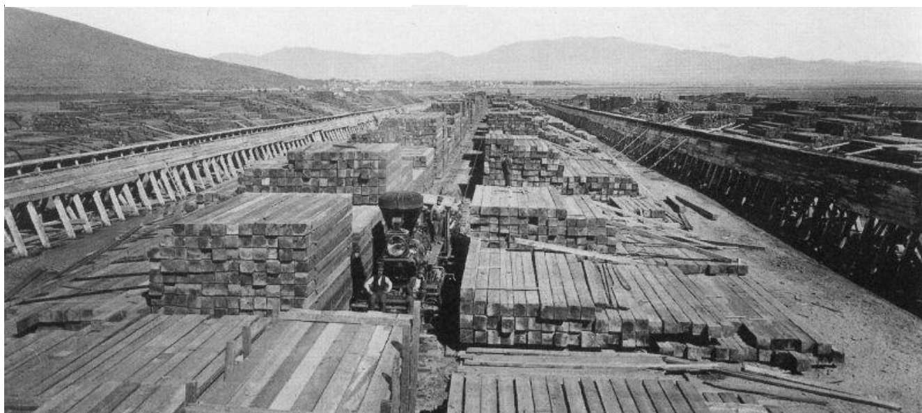
Lumber yard in Carson City at the terminus of the Clear Creek Flume
