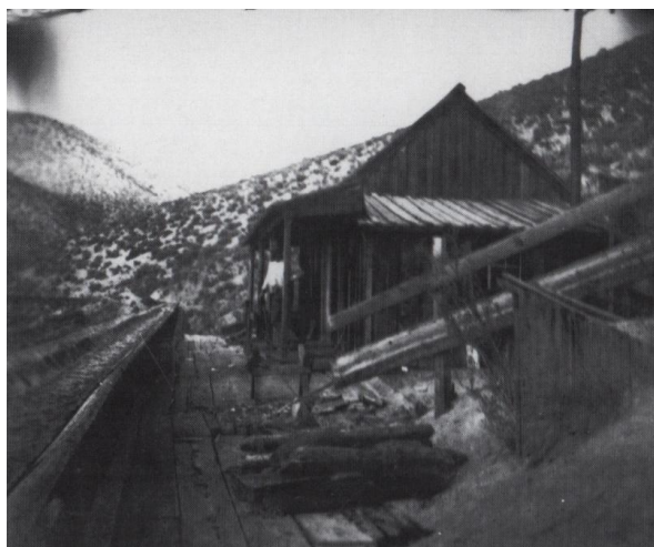
Flume shacks housed Chinese flume tenders
